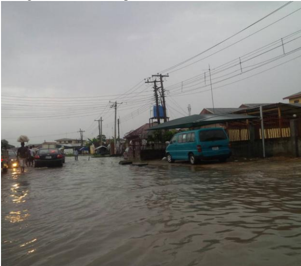
Plate 2: Nkpolu Road 1, Rumuigbo
