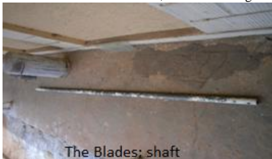
Figure 9: The Blades shaft Constructed
