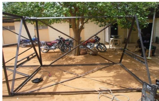
Figure 12: constructed triangular cage for blade housing
